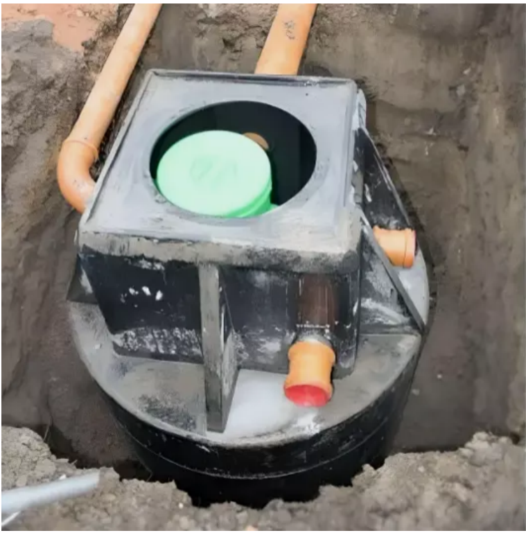
Aquatrio filter and adjoining pipework
